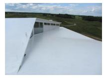
waterproofing membrane (without joints or overlaps), of high mechanical and external resistance, thermoset and elastomer (with the ability to bridge the possible fissures of the support). The coating, once cured, is inert, free of hazardous materials and heavy metals, making it fully recyclable at the end of its useful life. The membrane heals in a few seconds and its commissioning is in a few hours.
